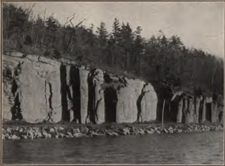
A. INTERSECTING SERIES OF PARALLEL AND VERTICAL FISSURE (JOINT) PLANES IN ROCK EXPOSED ON THE SHORE OF CAYUGA LAKE NEAR ITHACA, NEW YORK. (After a photograph by Tarr.)
